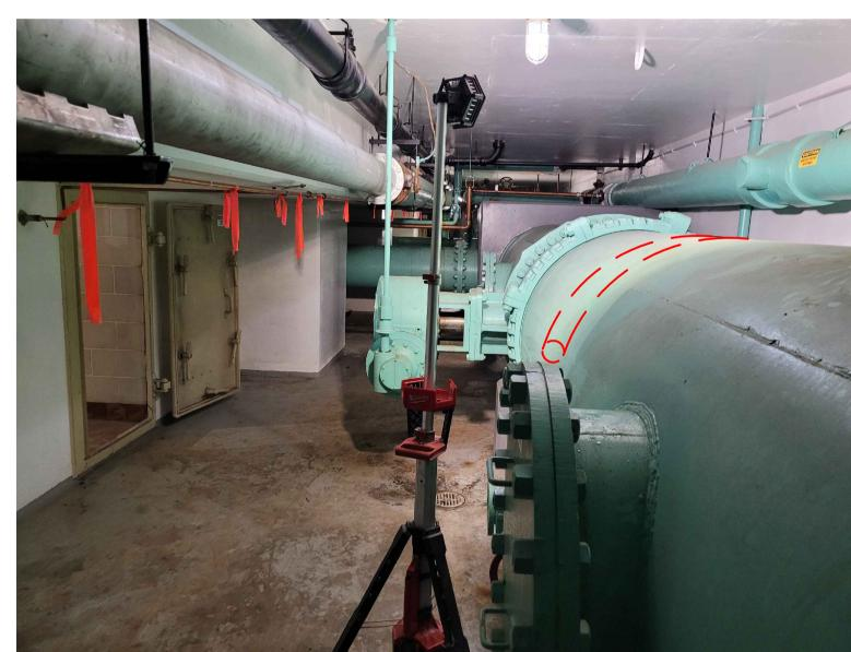
**PROPOSED LOCATION OF FPI MAG-METER (FE-M1531) LOOKING SOUTH (HORIZONTAL INSTALLATION)**
